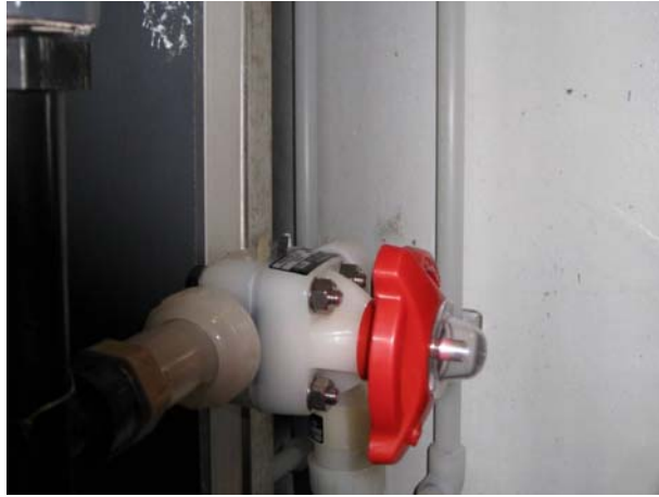
PVDF Diaphragm Valve for isolation
